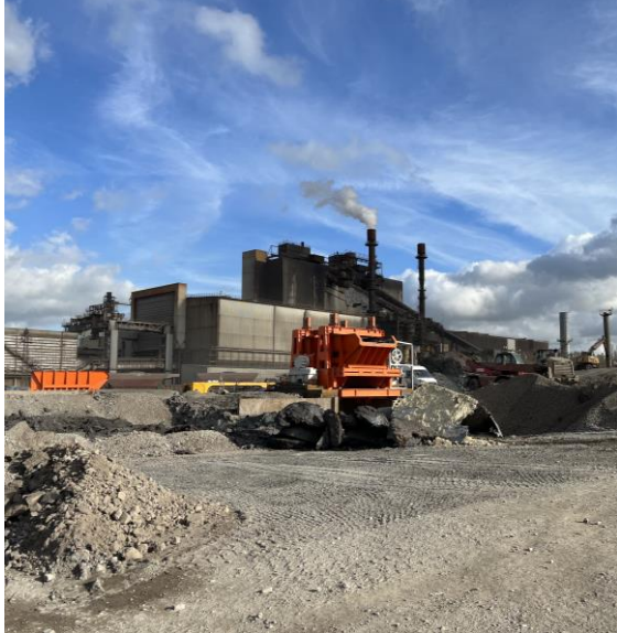
Outside area of the steel plant, HBM, Hot Box and the tipping device
